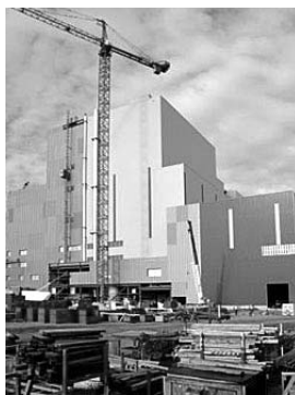
The outside façade of Weston 4 is taking shape.
